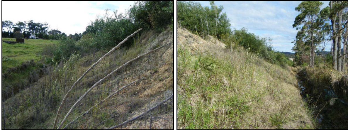
View of batters looking Northerly and Southerly direction - June 2009
