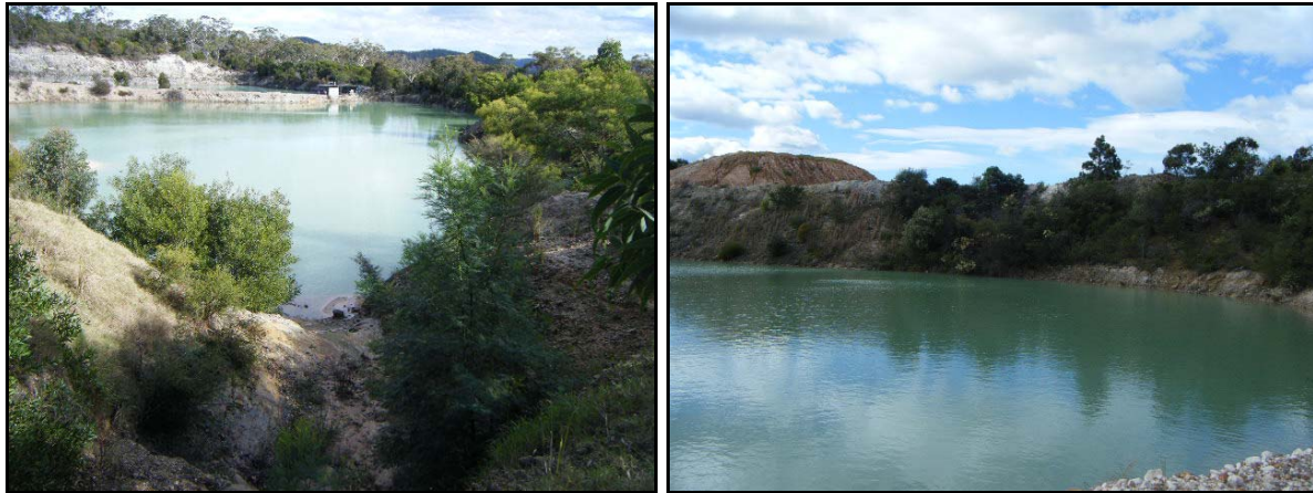
Alternate views of lower containment dam and surrounds
