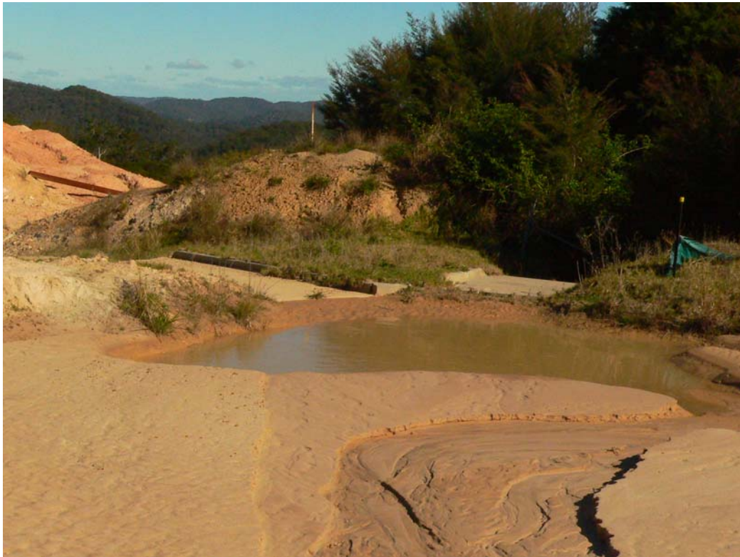
Photo sediment dam water sharing weir
