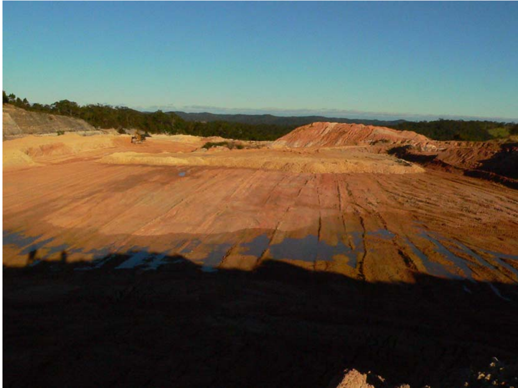
Photo capped cell 4 and 5
